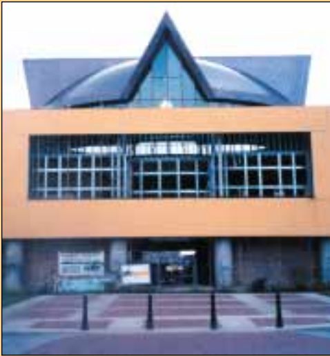
The new Tubman African American Museum, currently under construction, on Cherry Street
